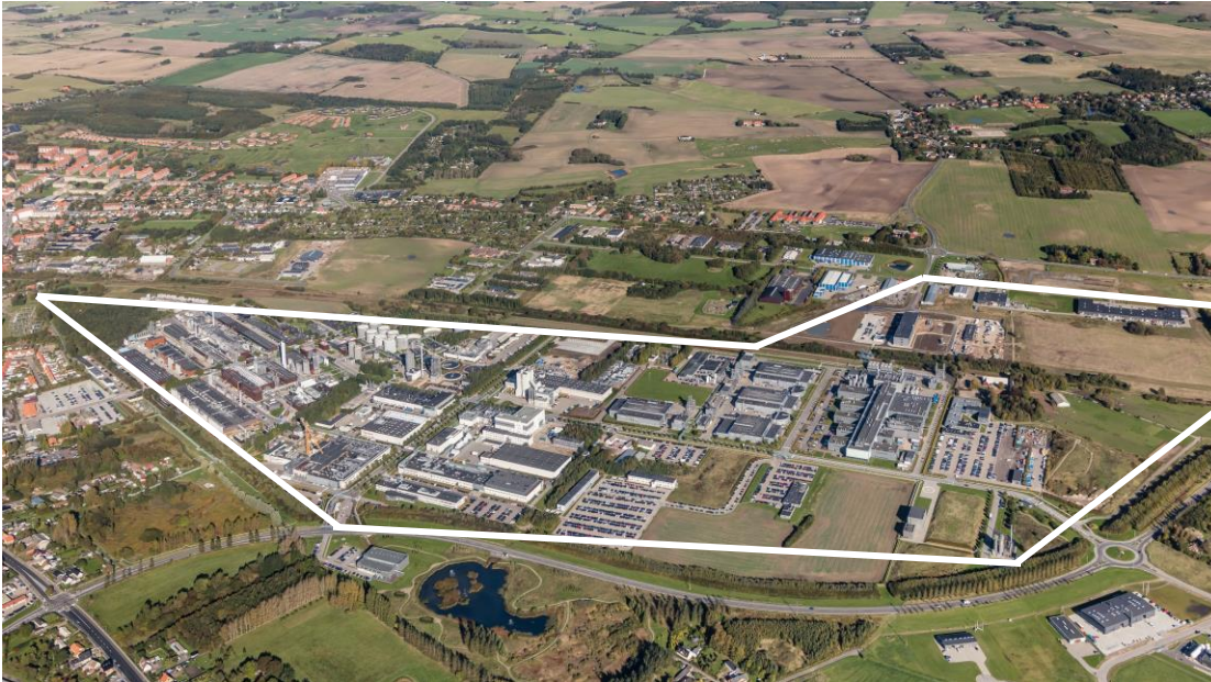
Site Kalundborg around last CMD
